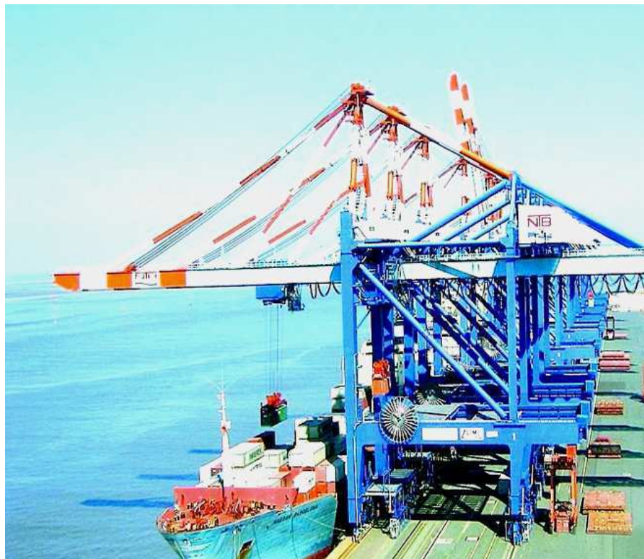
Figure 3.1: Port crane: container crane
